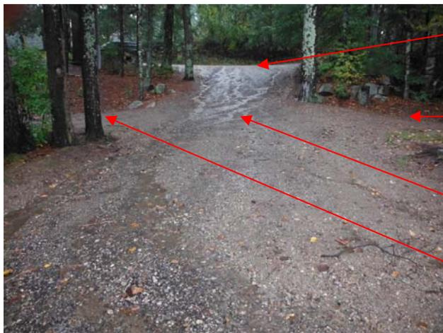
Install an open-top culvert across top of the ramp to catch precipitation and runoff water from roadway. Direct the runoff water north into a stone-filled drywell placed into the wooded area.
